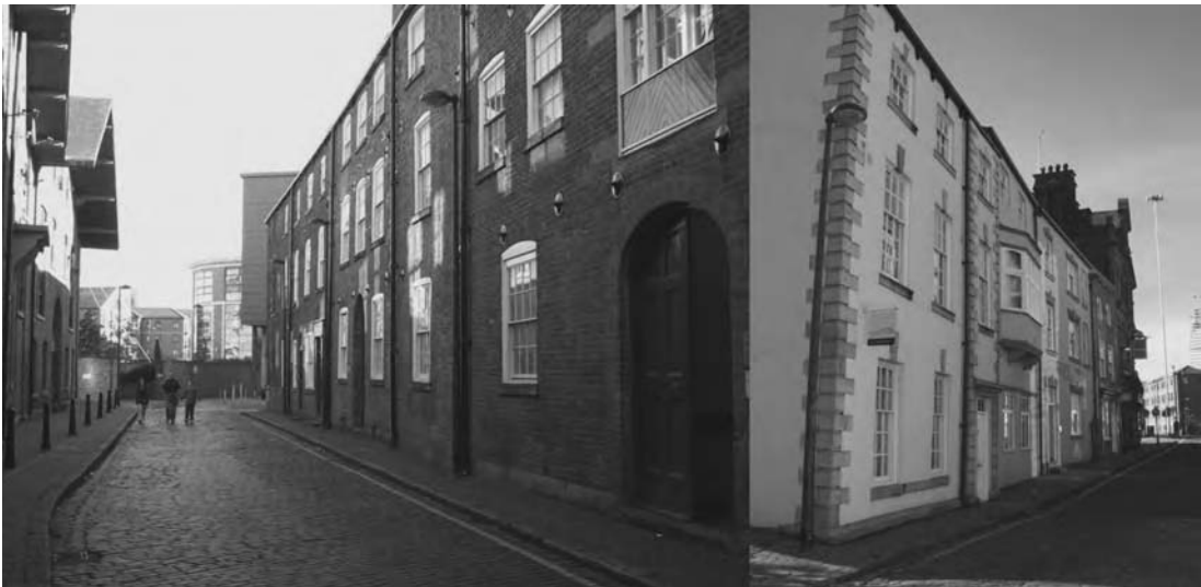
7.4 Sense of place overlooked by later development phases south of the Aire river
