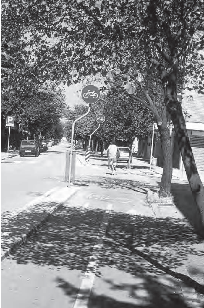
Fig. 51.2 The most common cycle routes in existing streets are the result of a reduction of the carriageway, often reducing motor traffic to one-way and reshaping parking. Cyclists are protected by a continuous line of twin concrete kerbs or by raising the cycle route.
