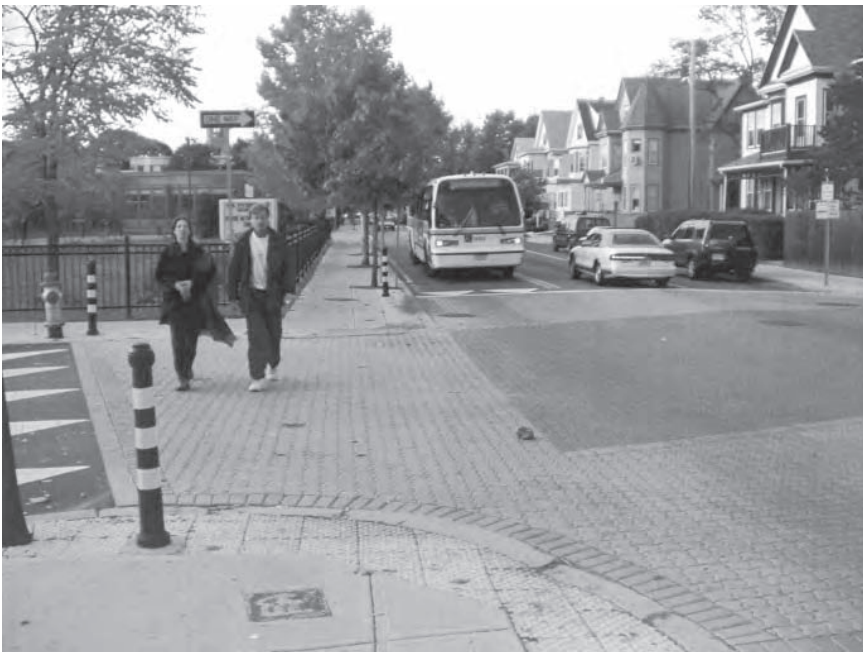
Fig. 46.2 Raised intersection in front of a school.
