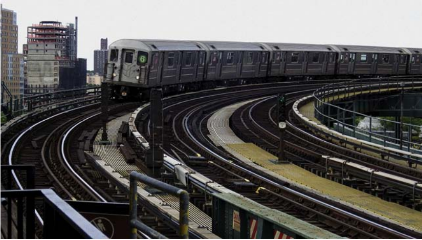
FIGURE C.32 Number 6 Train on elevated track curve. Photo courtesy of Joe Raskin, http://wanderingnewyork.tumblr.com/ .
