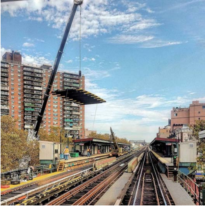
FIGURE C.28 Construction on elevated track. Photo courtesy of Joe Raskin, http://wanderingnewyork.tumblr.com/ .
