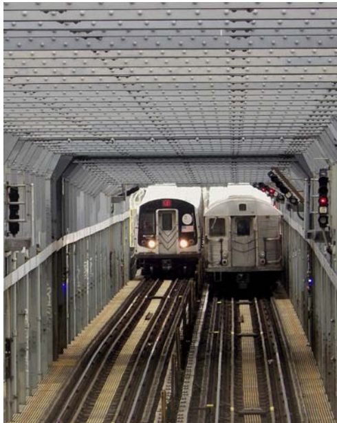
FIGURE C.21 Trains passing each other on Williamsburg Bridge. Photo courtesy of Joe Raskin, http://wanderingnewyork.tumblr.com/ .
