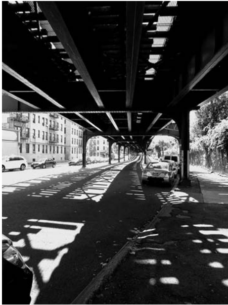
FIGURE C.8 View beneath elevated train structure. Photo courtesy of Joe Raskin, http://wanderingnewyork.tumblr.com/ .
