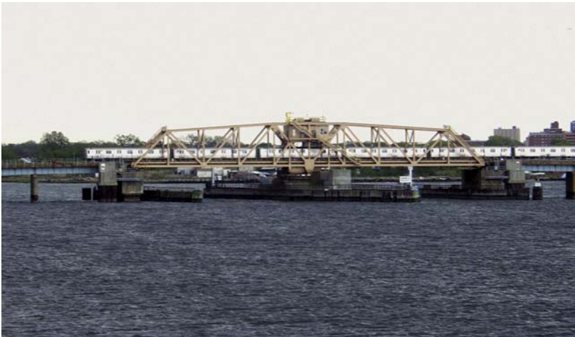
FIGURE C.5 A Train on Jamaica Swing Bridge Flushing Bay. Photo courtesy of Joe Raskin, http://wanderingnewyork.tumblr.com/ .
