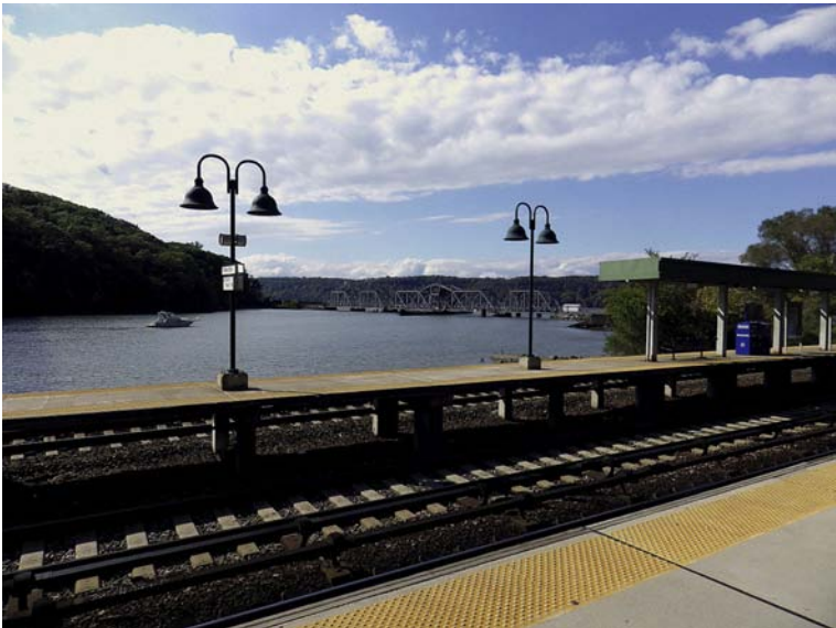
FIGURE C.31 Metro-North Hudson Line station platform with bridge in background. Photo courtesy of Joe Raskin, http://wanderingnewyork.tumblr.com/ .
