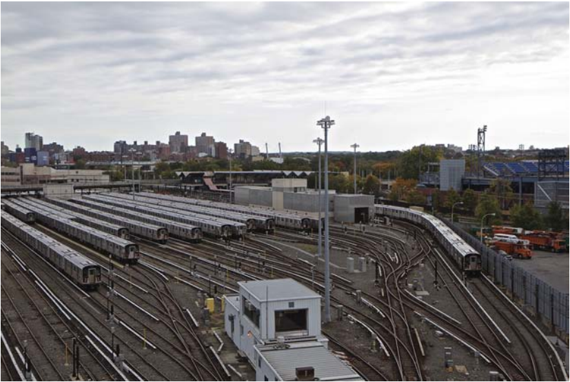
FIGURE C.27 Corona Train Storage Yard. Photo courtesy of Yekaterina Aglitsky.
